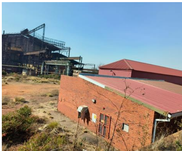
Photograph 2-5: Northeastern view of the electrical substation
