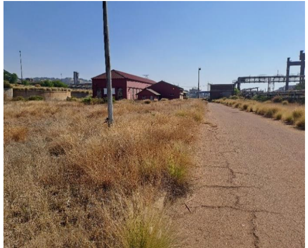
Photograph 2-10: Western view of all the buildings on-site.
