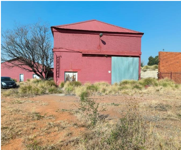
Photograph 2-3: Eastern view of the site with building infrastructure.
