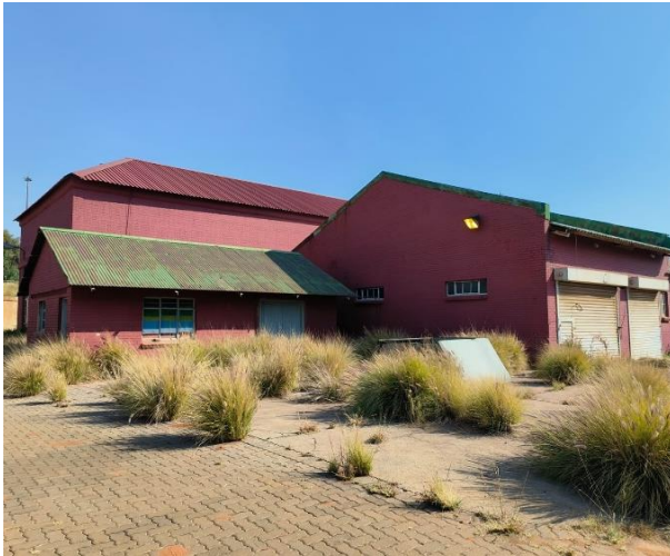
Photograph 2-1: Southwestern view of the second and third buildings (middle portions of the site).
