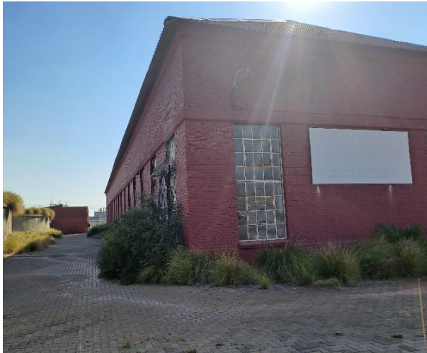
Photograph 2-9: Western view of the main building on-site.
