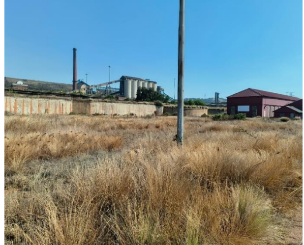
Photograph 2-4: Southwestern view of site.
