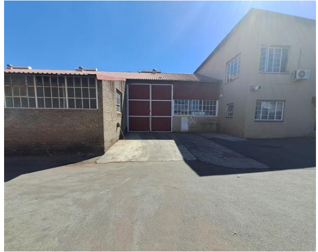
PHOTOGRAPH 3-2: South-western view of the facility – taken from northeast of the site.
