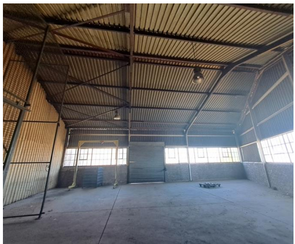
PHOTOGRAPH 3-6: Main factory entrance door. Picture showing the factory main floor.
